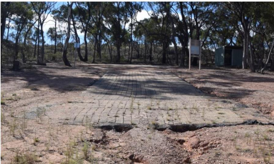
**Figure 7.3 Existing boat ramp cracking and erosion.**
