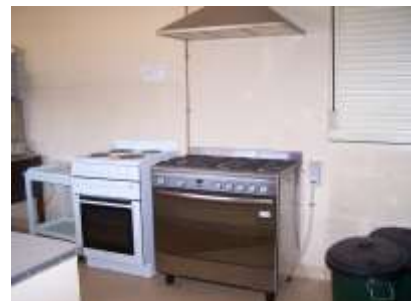
The new oven for the Hall kitchen
