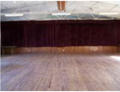
The Hall before
