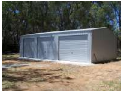
The new machinery shed
