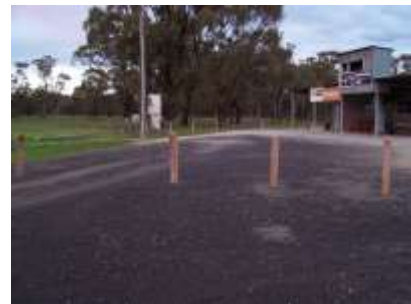
Bolards to divert traffic from in front of the Clubrooms
