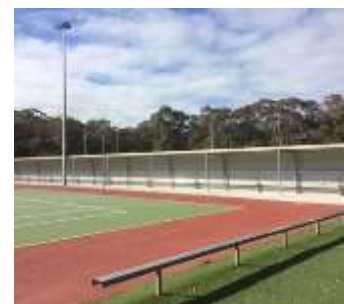
New Shelter Netball & Tennis courts
