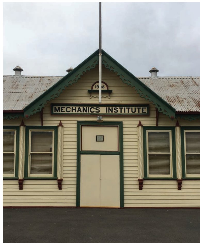
Mechanics Institute Hall, Main Street Korong Vale.
