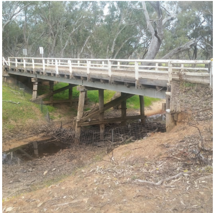
Sloans Road Bridge.
