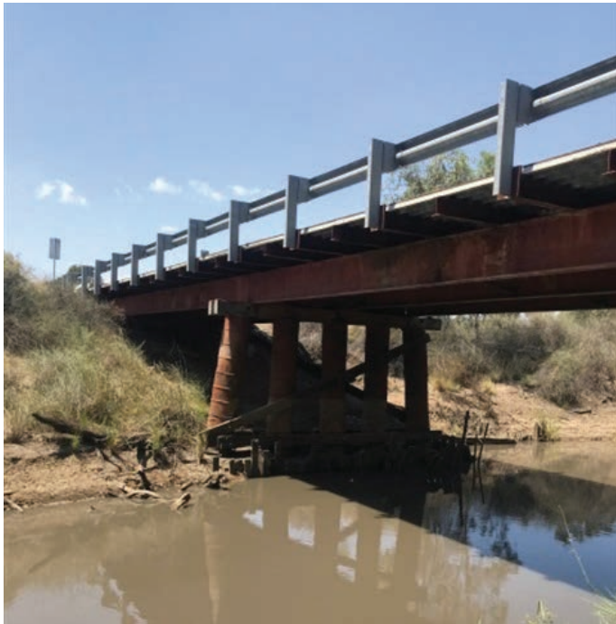
Appin South bridge.
