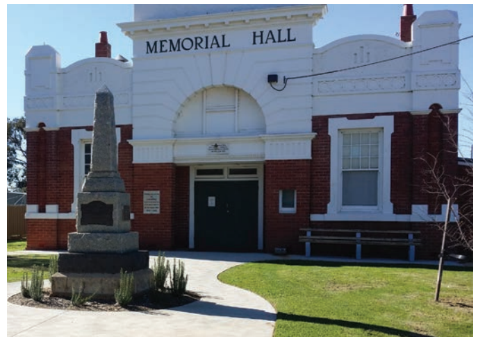
The Pyramid Hill Memorial Hall received $10,000 towards the installation of reverse cycle air-conditioning units as part of the 2018/19 Community Grants Scheme.
