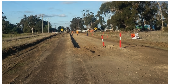
Flood restoration works in progress at Tandarra Serpentine Road.
