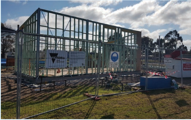
New changerooms under construction at the Inglewood Swimming Pool.
