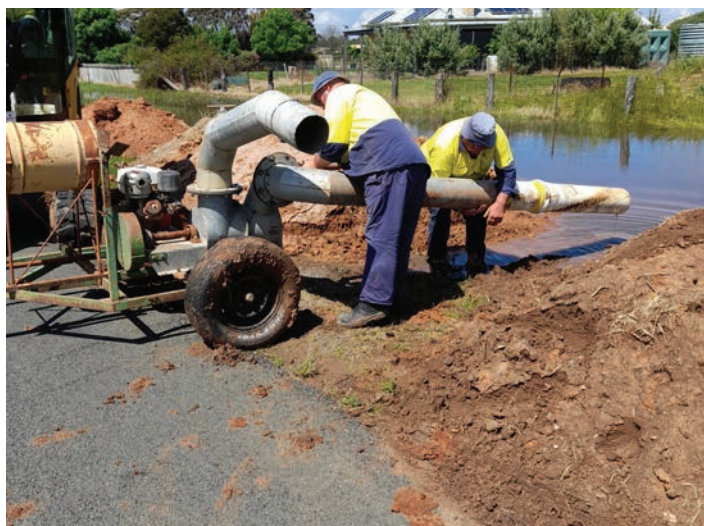
Flood works taking place in October 2022.
