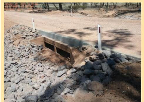
Old Boort Road at Woolshed Flat before (top image) and after flood recovery works (above). The works included beaching and installation of concrete edge beams.
