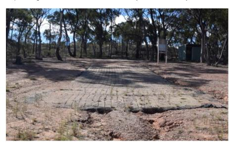
Figure 7.3 Existing boat ramp cracking and erosion.
