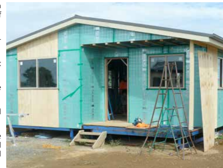
The new house under construction in Shepparton.
